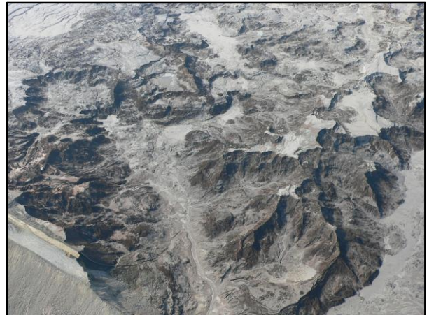
The breach at the Mount Polley tailings pond. For scale, see the bulldozer in the bottom left-hand corner.
