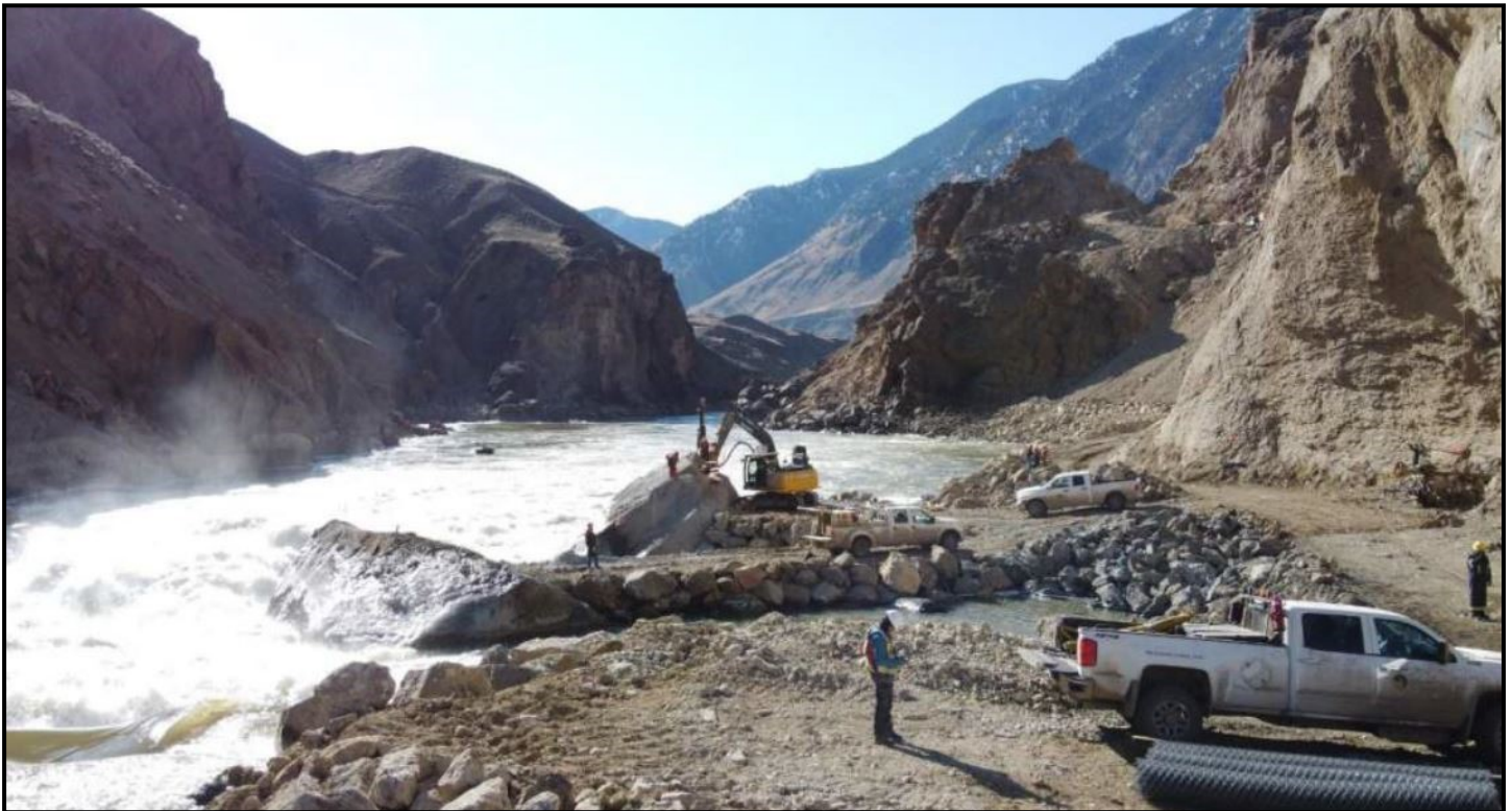
PICTURED: Crews drill boulder H7 in preparation for blasting
