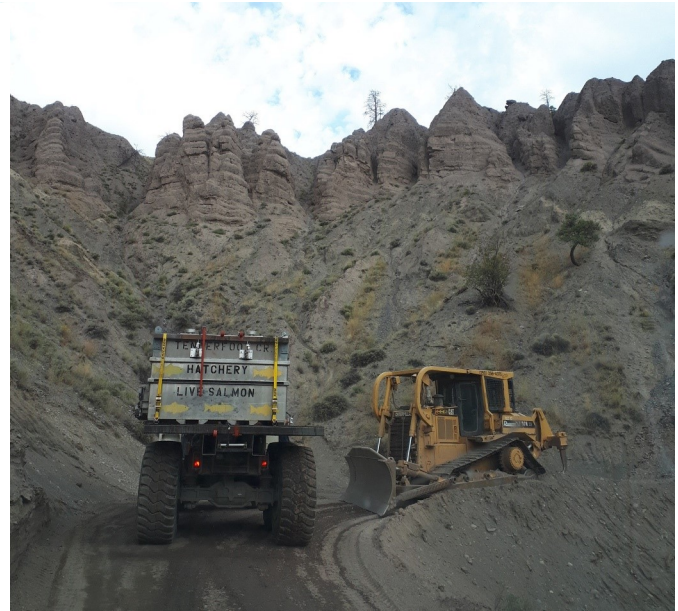
The truck outfitted with a fish holding tank to transport salmon by road upstream of the slide.
