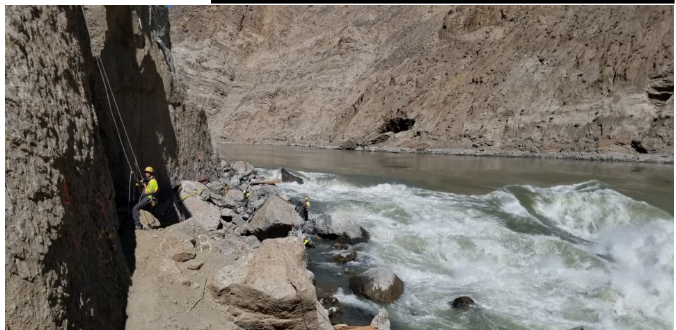
Rock scalers work at river level to manipulate rock.
