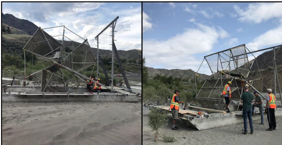
The Fish Wheel being assembled on site.
