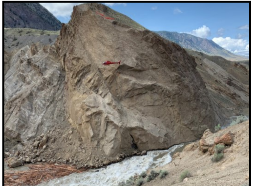
Figure 1. Scaler crews working on the cliff face as a helicopter passes.
