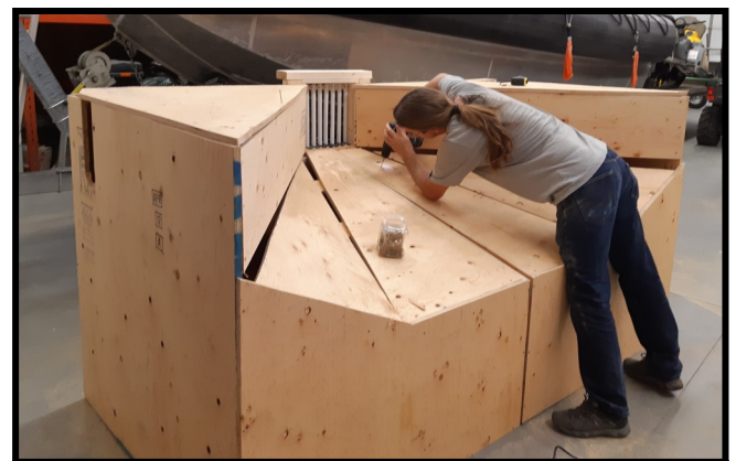
Figure 2. The fish weir being built for the holding pond.
