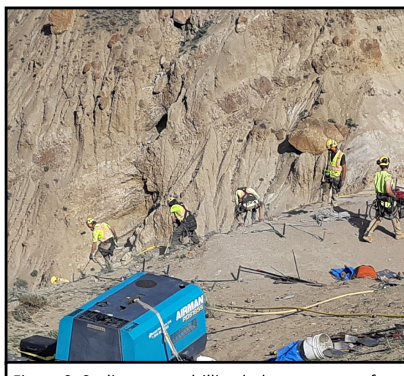
Figure 2. Scaling crews drilling holes to prepare for the controlled blasting operation.
