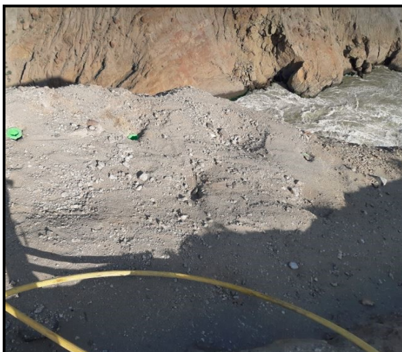
Figure 1. Holes drilled by scaling crews.
